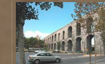
Valens Aqueduct 348 A.D.
